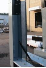
*D. Top Corner Diagonals* - These are two flat bars with pre-drilled holes used to square up the sign. They are to be attached to the upper left and right corners of the sign. On signs over 10'6" tall they are packaged with the Side Frames when the Side Frames are shipped separate from the tops. On signs 10'6" and under they are pre-installed at the factory.
