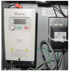
lead wires that match the existing wires. Remove the existing Inverter. New mounting holes may have to be drilled for the new Inverter. We typically mount replacement Inverters with self taping screws. Connect the wires on the Inverter wire for wire. Remove one lead wire from the new Inverter and replace it with the permanent wire.
