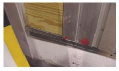
Measure the center-to-center distance of every few louvers to ensure consistent 6" spacing. Measure from jig extrusion #1 across the total distance of the jig to ensure proper spacing.
